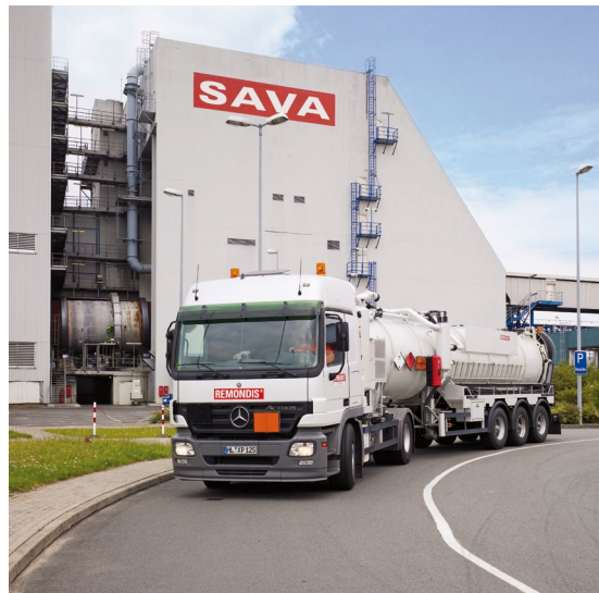
The hazardous waste incineration plant owned by SAVA GmbH & Co. KG – one of the many internationally active companies belonging to the REMONDIS Industrie Service Group
