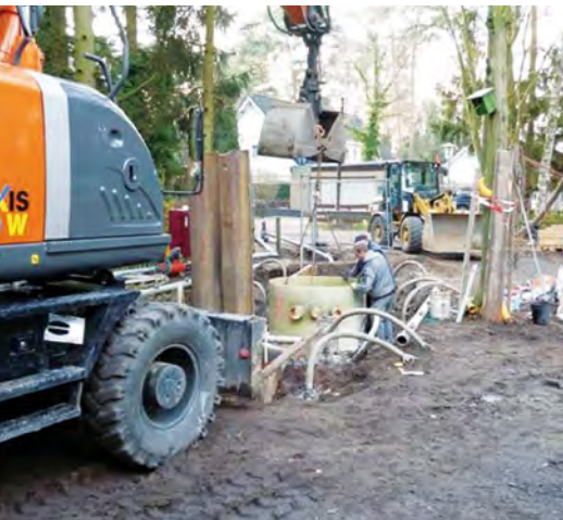
Construction work being carried out on a new pump station
