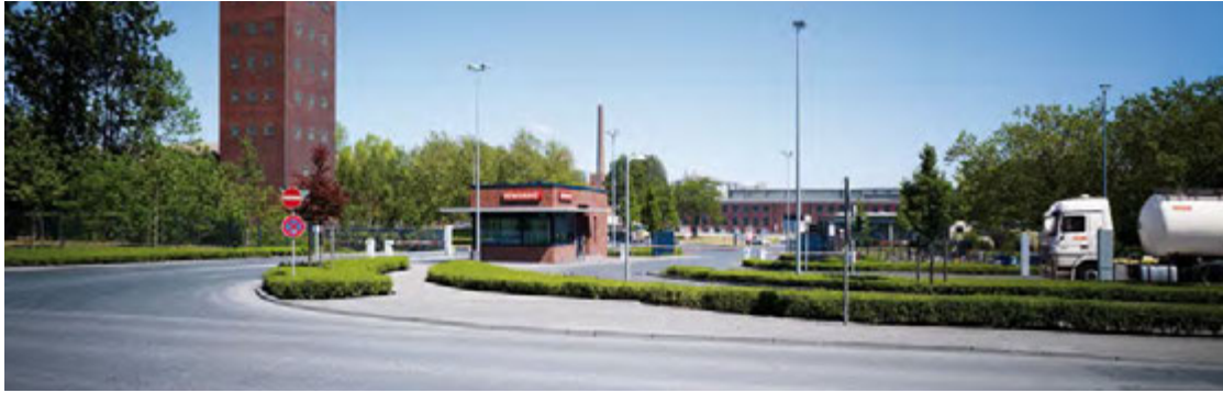
The REMONDIS Lippe Plant has a well-developed on-site infrastructure and excellent connections to all different forms of transport
