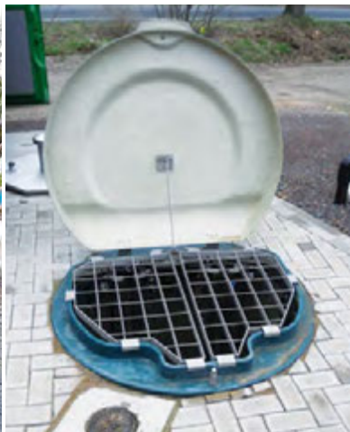
The pump stations have been installed below ground
