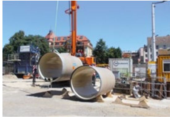
The newly laid pipes are truly impressive with an outer diameter of 1.72 metres
