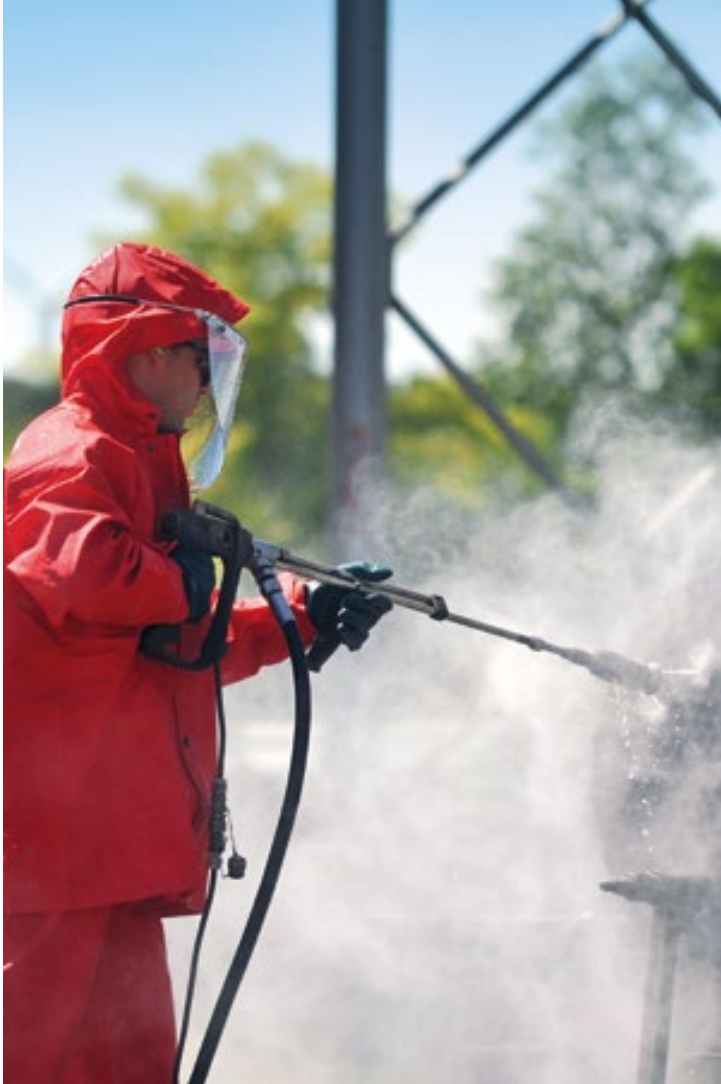
One of the employees in Schwedt demonstrated how a heat exchanger should be cleaned with a high pressure water jet
