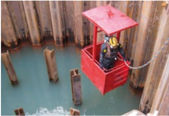
The section of the main sewer system that is being renovated in Cottbus lies 7 metres below the ground
