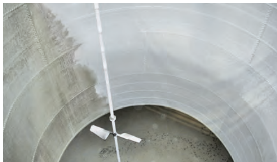
After: XERVON Oberflächentechnik coated the twelve-metre tanks after REMONDIS' subsidiary, BUCHEN, had removed all the deposits from the surface
